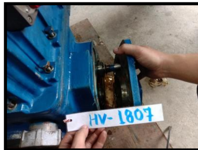
Fig 14. Inspect Shaft Hand Wheel
